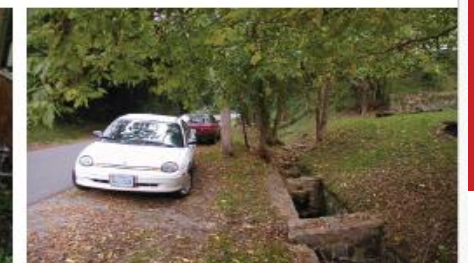
Keep historic culvert
